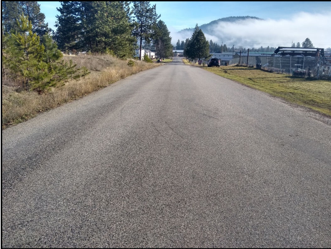
SITE PHOTO - 6: View from the west end of Aqua Avenue looking east.
