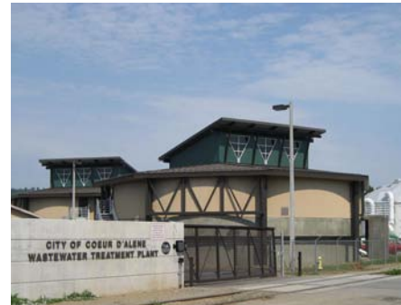
Wastewater treatment plant
