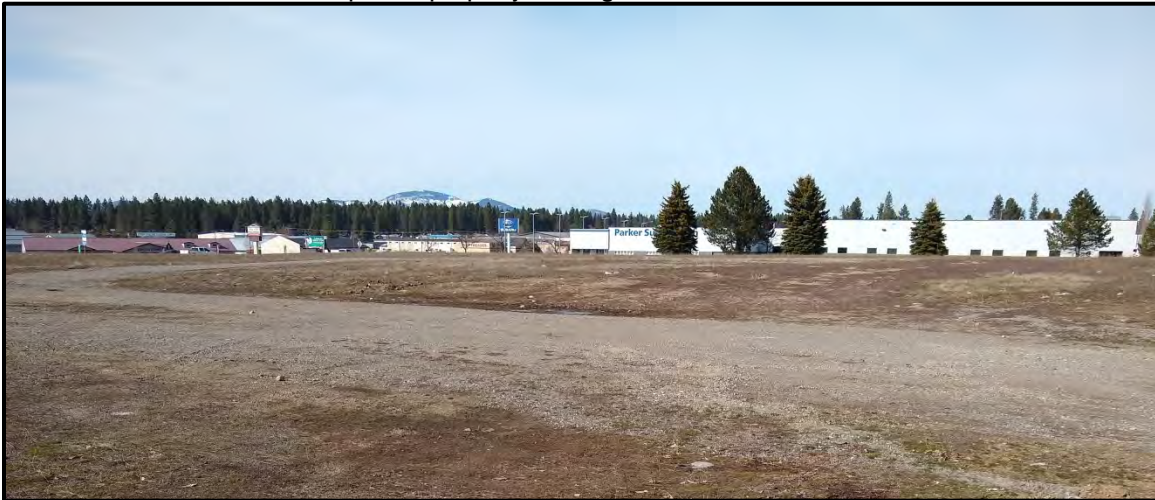
SITE PHOTO 5: East central part of property looking north.
