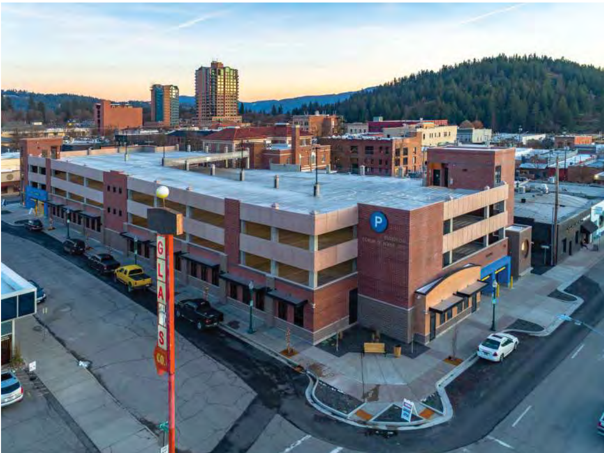
Parking Garage – 3 rd & CDA
