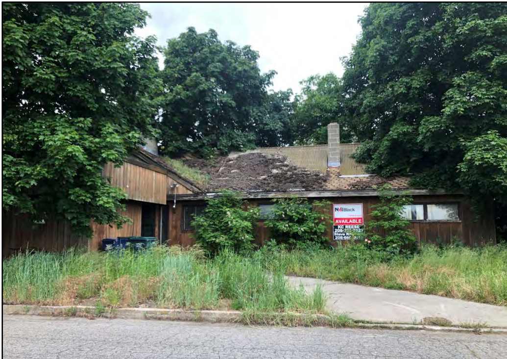
SITE PHOTO 2: View of the subject property along Cardwell Drive.
