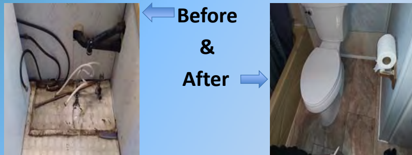
Subfloor repair and ADA toilet installed
