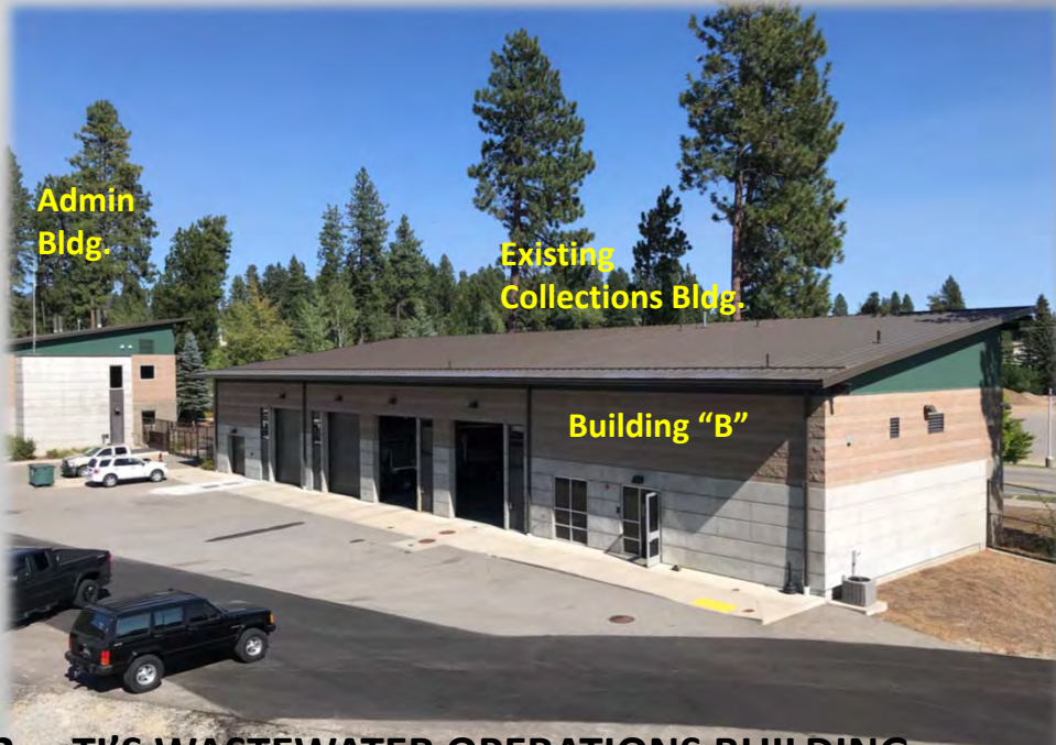
PHASE 2 – TI'S WASTEWATER OPERATIONS BUILDING
