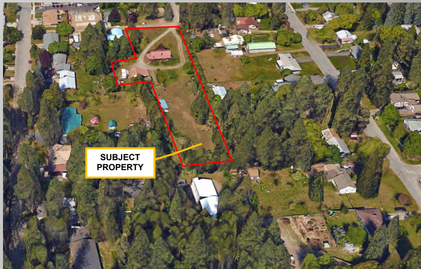
Bird's eye view of the subject property looking west
