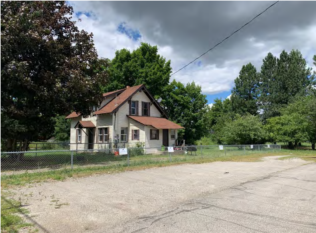
SITE PHOTO 2: View of the subject property facing northwest.
