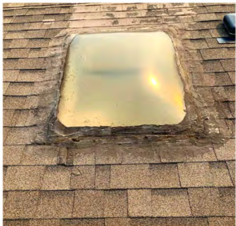
Leaking Skylight Removed and Roof Repaired
