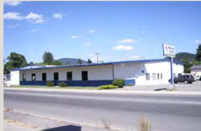
CDA SCHOOL DISTRICT MAINTENANCE BUILDING
