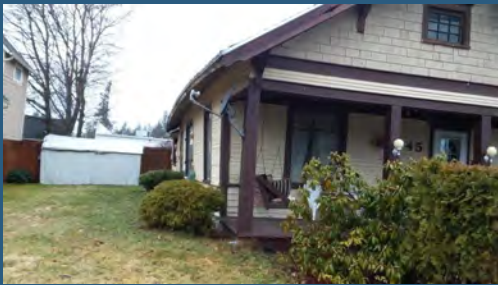
Wood foundation failing Truss and wall separation Demolition completed July 2022
