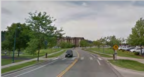
Centennial Trail Crossing
