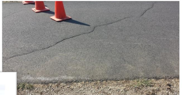
Repaired Broken Section of Trail
