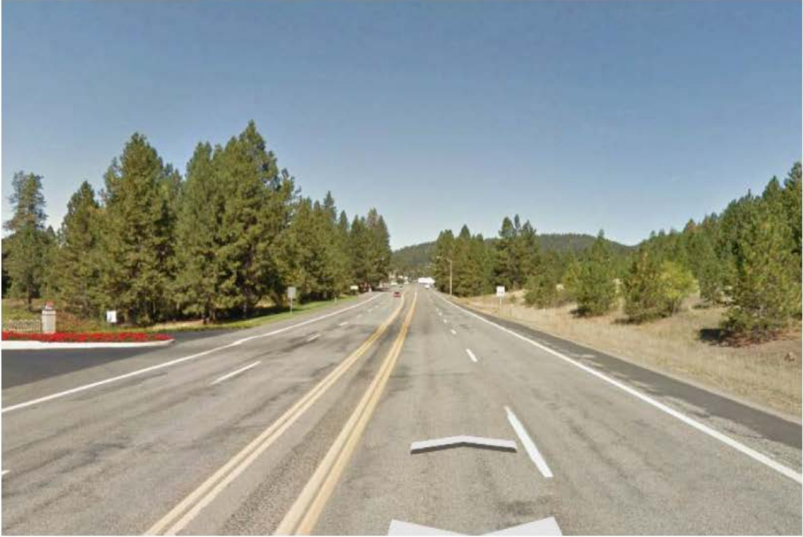
Figure 10 CDA Lake Drive Looking North-Before
