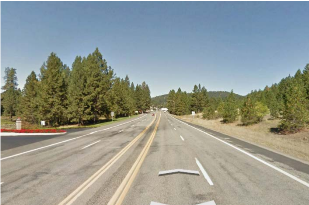
Figure 8 CDA Lake Drive Looking North-Before
