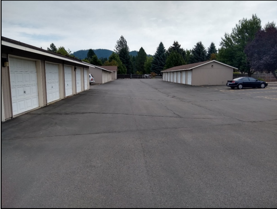
SITE PHOTO 5: Central part of property looking east.
