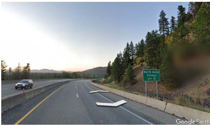
Figure 20 I-90- West Bound near Potlatch Hill Road - Before
