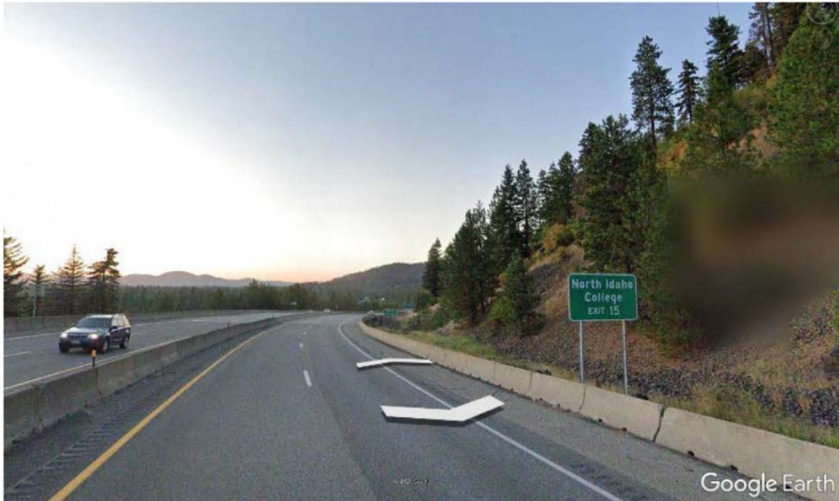
Figure 22 I-90- West Bound near Potlatch Hill Road - Before
