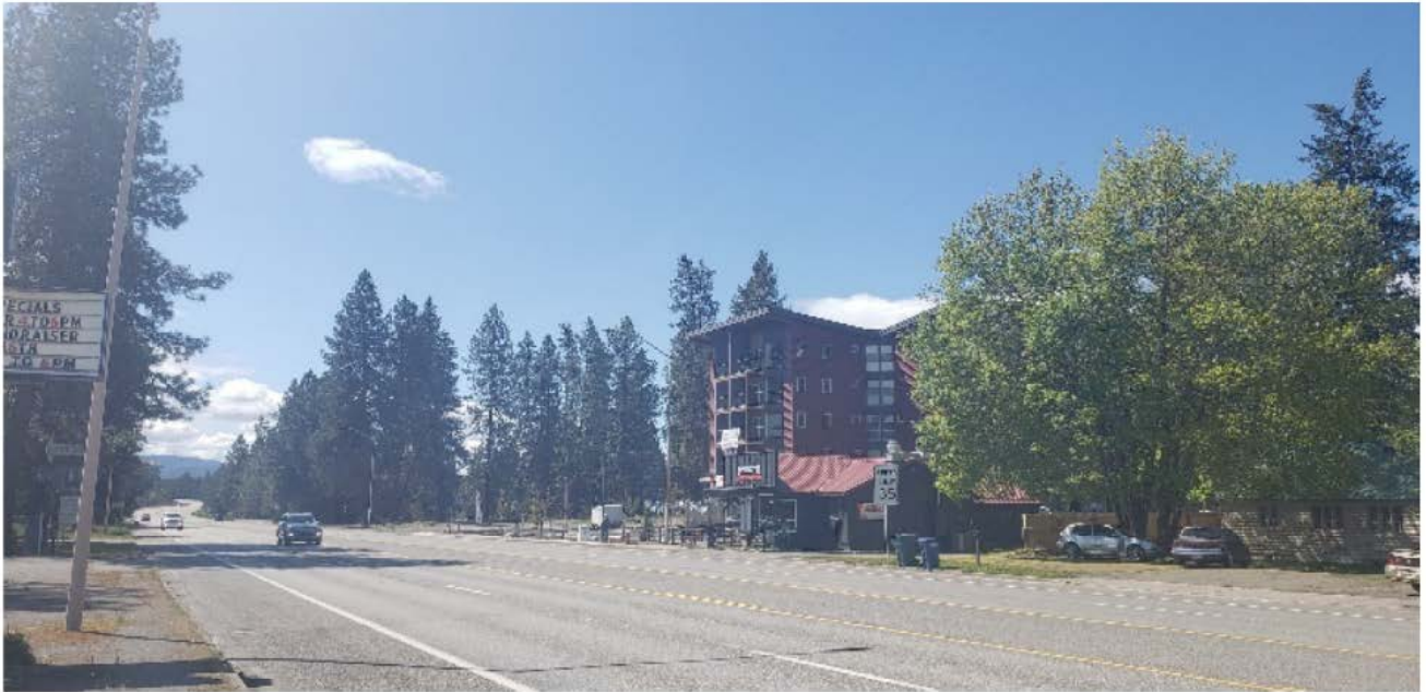
Figure 16 CDA Lake Drive Looking Southwest - Before
