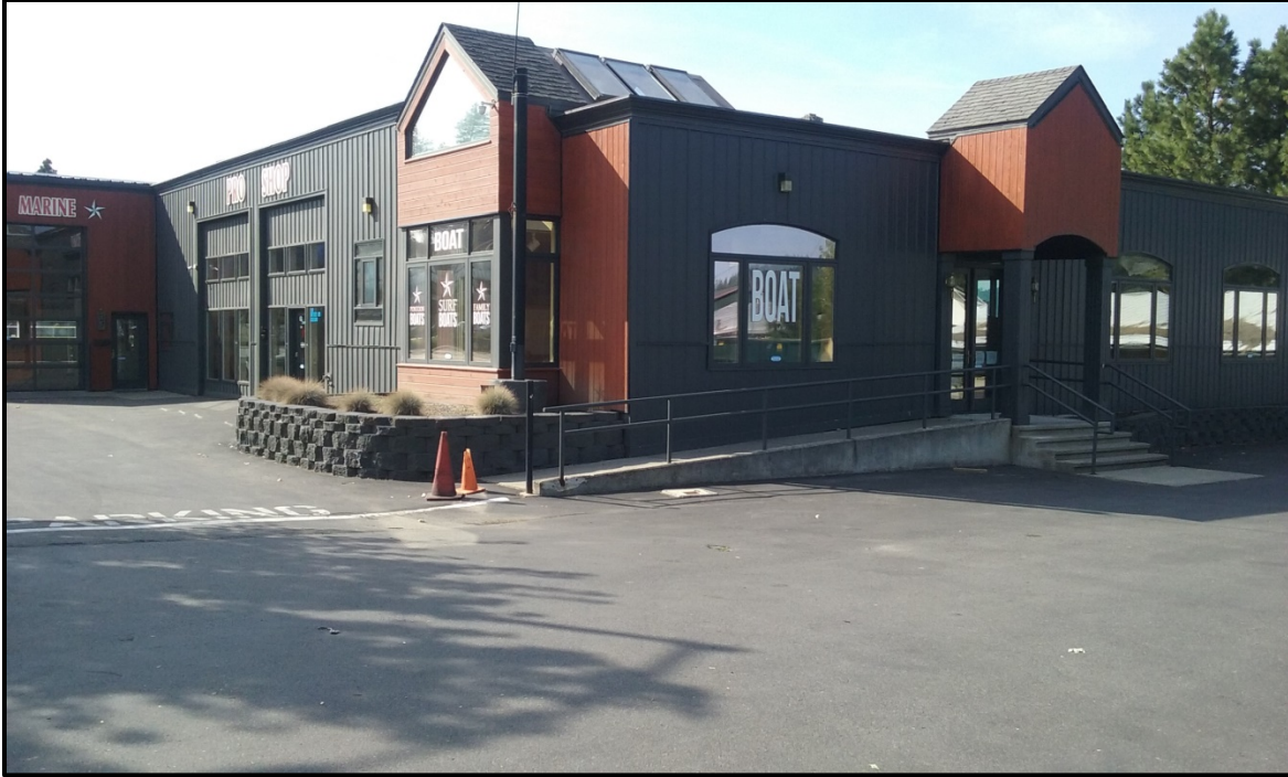
SITE PHOTO - 4: View from the northeast part of property looking southwest at the existing building.
