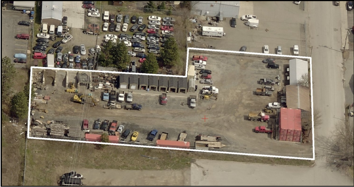
BIRDSEYE VIEW AERIAL PHOTO 1:
