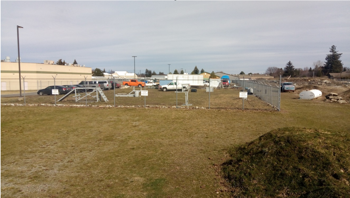
SITE PHOTO - 4: View from the southeast looking north.
