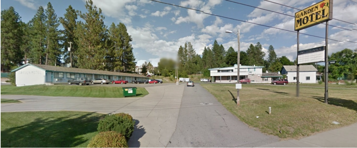
Site Photo – 1 Google Maps Street View from Northwest Boulevard looking east
