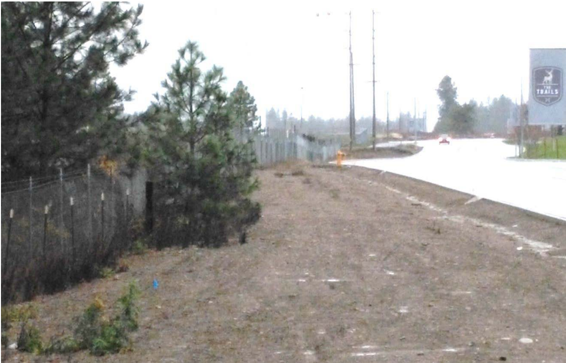
"Pinch point" along Hanley Ave.:
