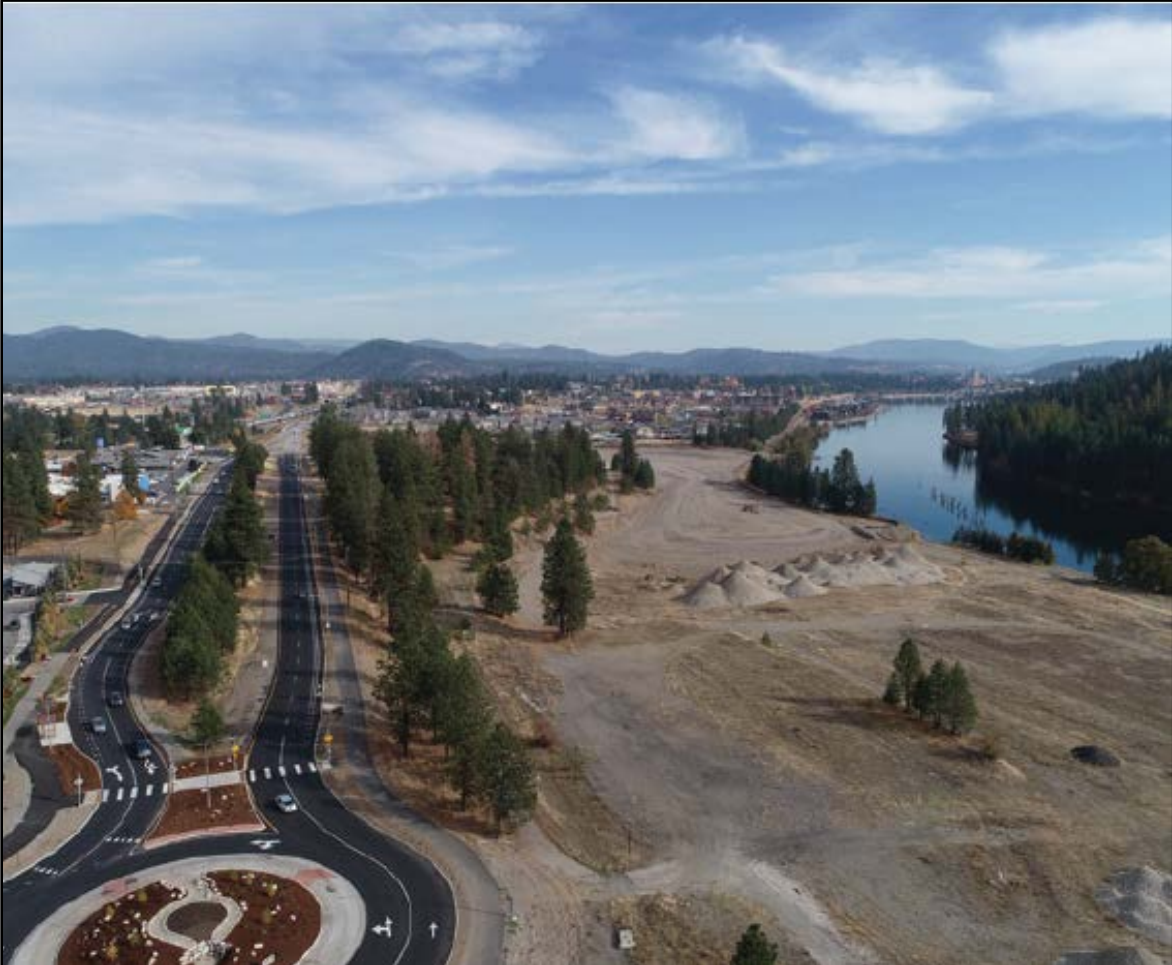
DRONE PHOTO FROM ATLAS ROAD & SELTICE WAY ROUNDABOUT
