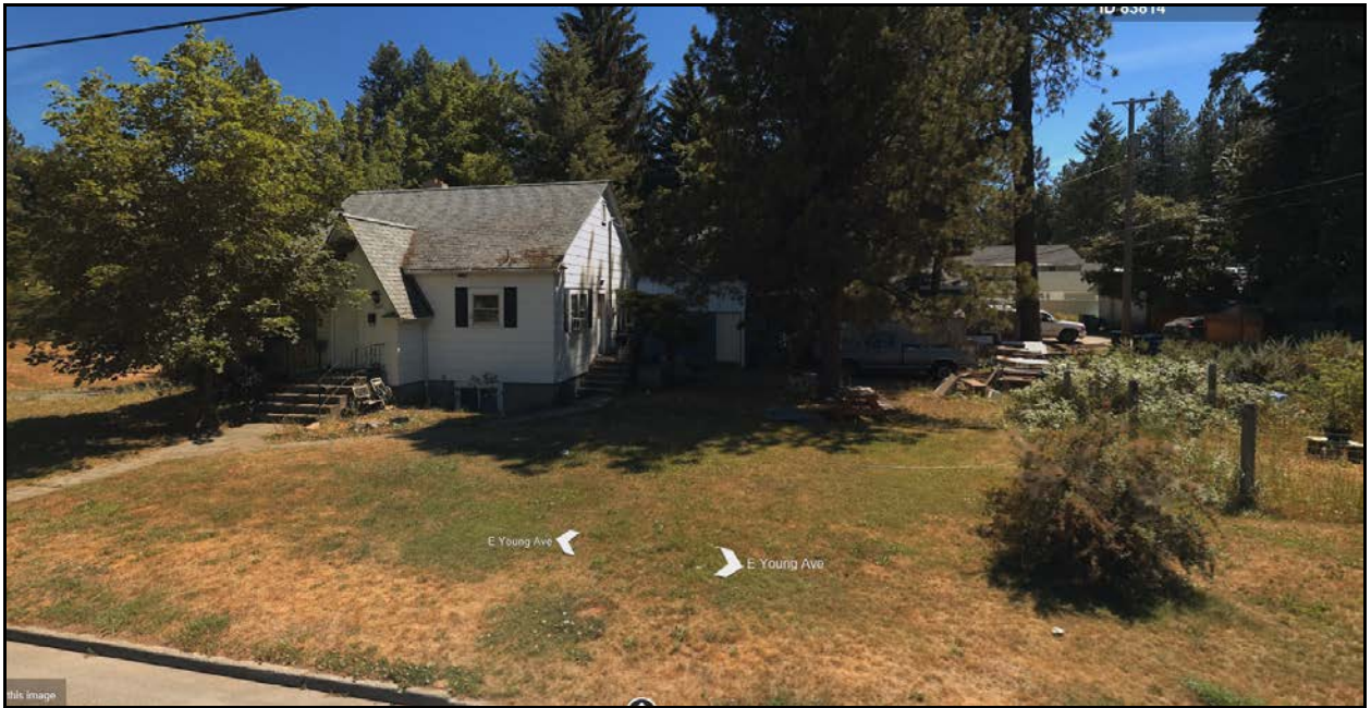
Looking south on Young Avenue at the single-family prior to +/- 3900 sq. ft. addition currently under construction.
