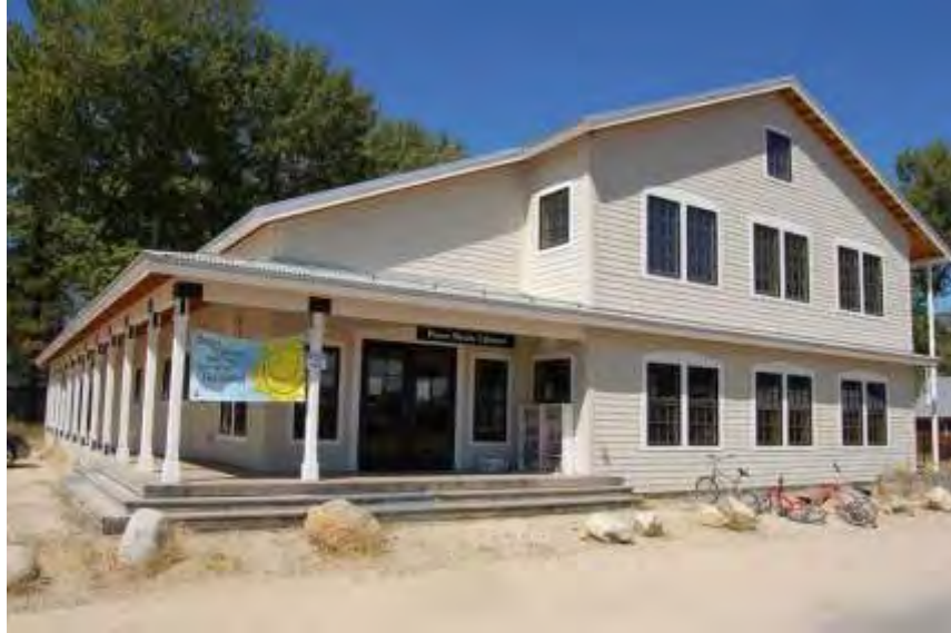
The Boise Basin Public Library, an excellent example of new construction in the Historic District featuring a boardwalk, shiplap siding, and multipane windows.
