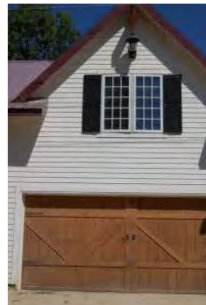
Figure 18. Good example of an appropriate wood-panel garage door.
