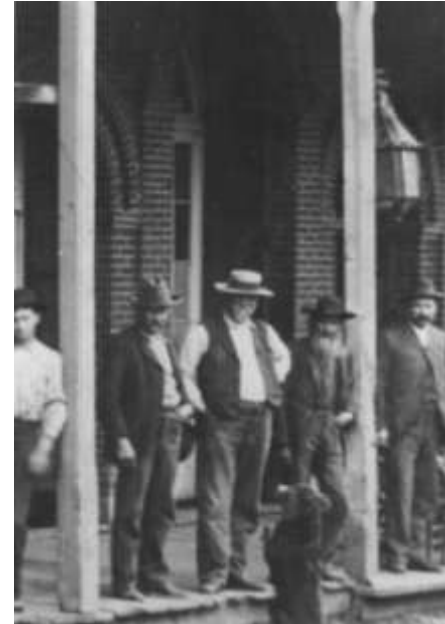
Figure 24. Kerosene lantern hanging in front of the Miner's Exchange.
