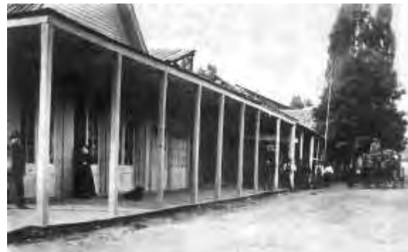
Figure 21. West side of Main Street looking north from Commercial Street. Notice milled posts.
