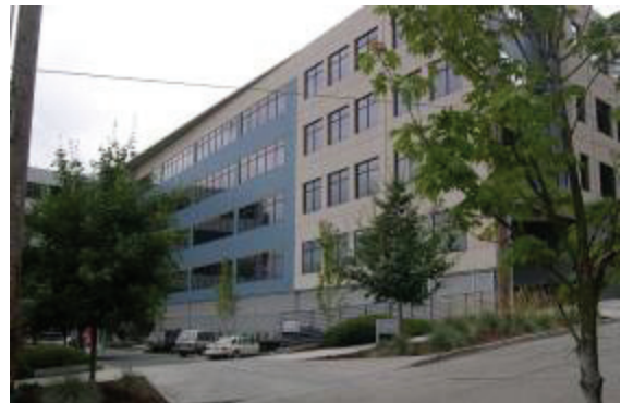
Parking Located Behind
