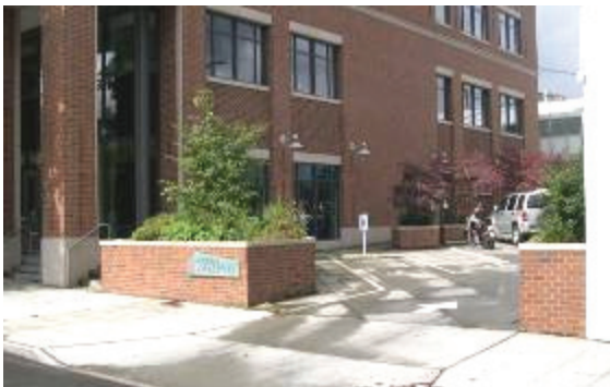
Parking Located To The Side
