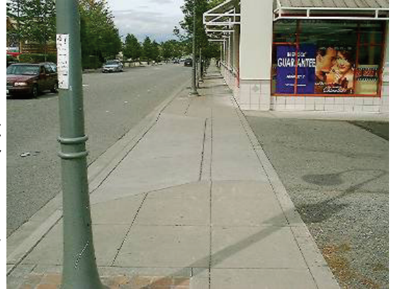
Sidewalk pavement is visibly continuous
